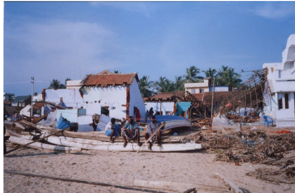
Collapsed houses at Kolachel village.
